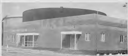
START AND FINISH POINT: Pictured is the new Reception Center which will be the starting and finishing points of the family tour program. Tour guests will gather at the Center for an introductory talk and upon completion of their tour through the refinery will be served refreshments here.
